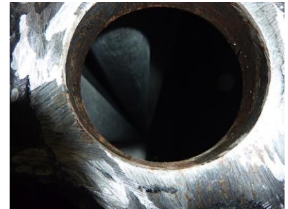
View inside the water drum (after)
