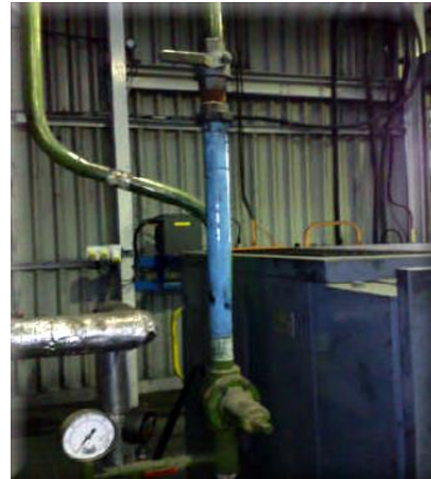
Columbian Chemical Installation
