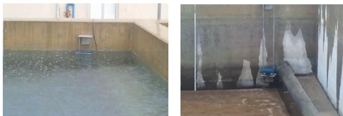
Figure 4: Left: LG Sonic Installed in Sand Filter. Right: When Filter is Empty it can be Seen that the Walls and Filter Medium are Kept Clean.
